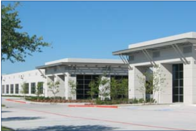
North Belt Office Center III & IV Houston, TX 107,200 SF Two, Single-Story Class "A" Office Buildings
