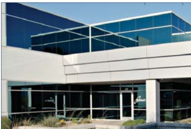
Foothills Corporate Centre II Phoenix, AZ 144,908 SF Two, Single-Story Class "A" Office Buildings
